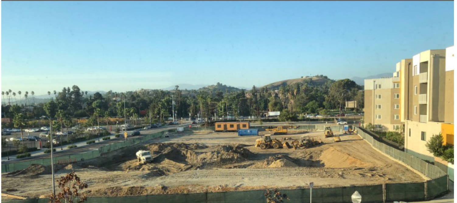
Construction of hotel project on land already owned by the university.
